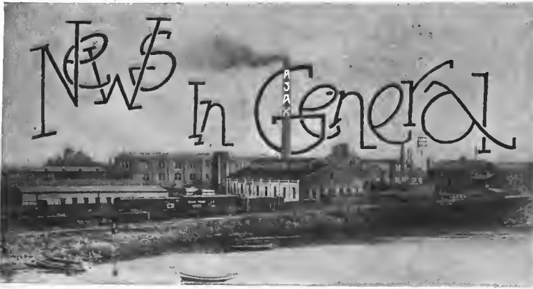
Factories of the Ajax-Grieb Rubber Company, at Trenton, N. J.
